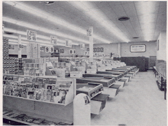
The checkstand area of LDD Store 96 as it appeared on opening day, May 22. Note the conveyor and baskets which are used instead of carry-out boys.
