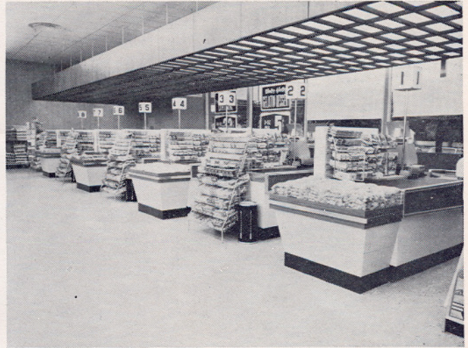
Lighting in the drop ceiling over the checkstands is unique, designed specifically for the new store. Illumination is bright but not glaring.
