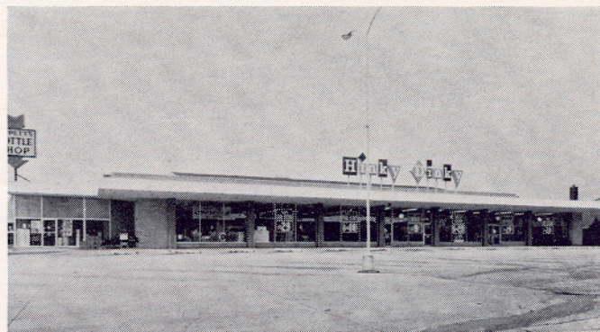
Store 52 shows its new face to the public. The sign was replaced, and even the lighting was modernized. Wide paneling along the over-hang improved the design.
