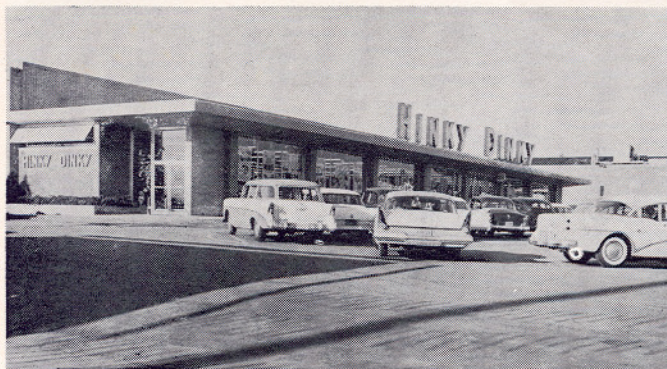
Store 52, the largest supermarket in the Hinky Dinky chain, as it appeared before it was completely remodeled. Note the old block-letter neon sign over the entrance.
